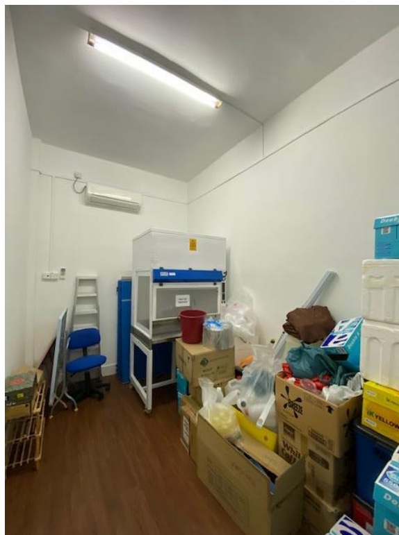
Figure 2: Installation of EV Sun germicidal lamp at store room.
